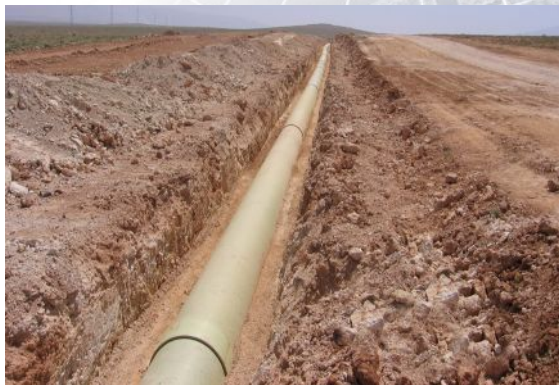
Installation of GRP and Carbon Steel Pipes
