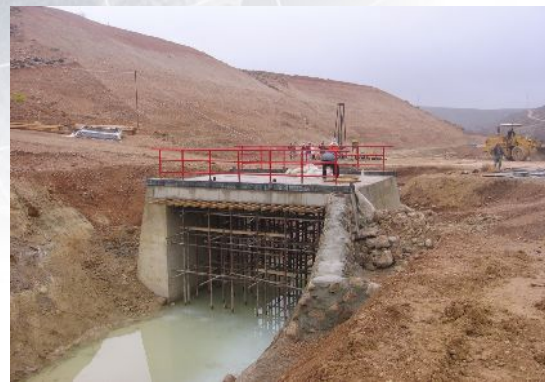
Construction Works - Package 1
