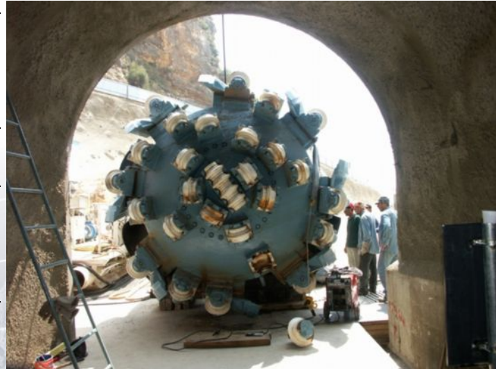
Cutter Head of the Tunnel Boring Machine
