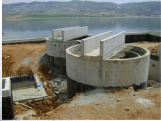
Clarifiers Construction at the Saghbine Wastewater Treatment Plant
